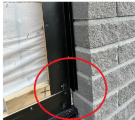
STARTER AND TRANSITION TRIMS FOR A FINISHING INSTALLATION IN BETWEEN ANOTHER TYPE OF CLADDING: MINIMUM SPACE OF 1/16".
